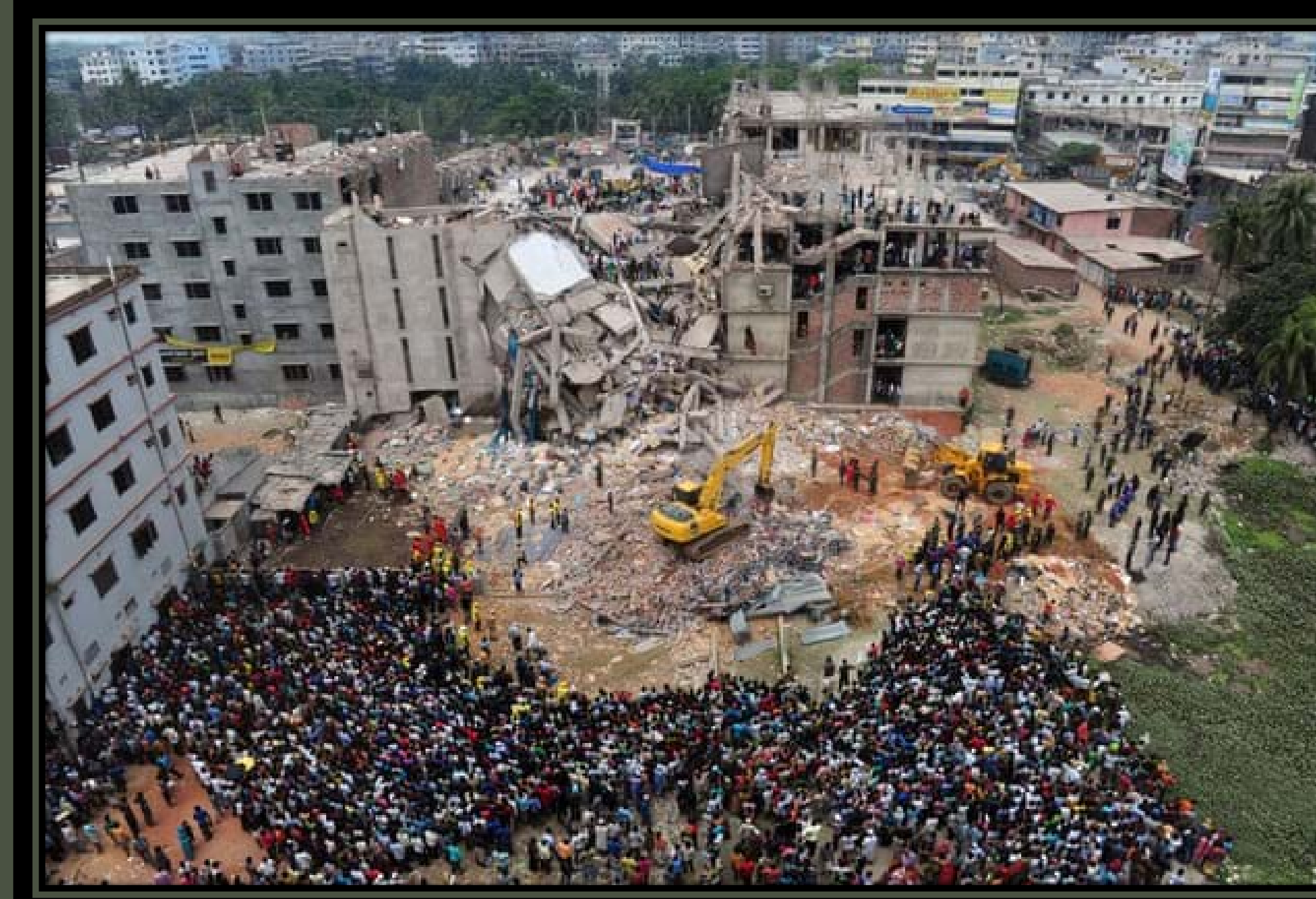
Figure 2: Aerial view of the Rana Plaza building site after it collapsed in April 2013, killing more than 1,100. Photograph: Munir Uz Zaman/AFP/Getty Images
