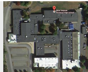
Aerial view of Wolcott Tech.
