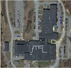
Aerial view of Grasso Tech.
