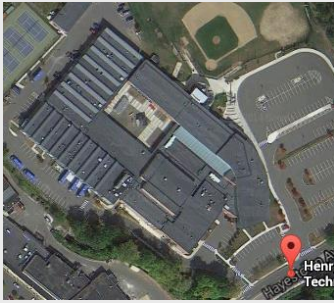
Aerial view of Abbott Tech.
