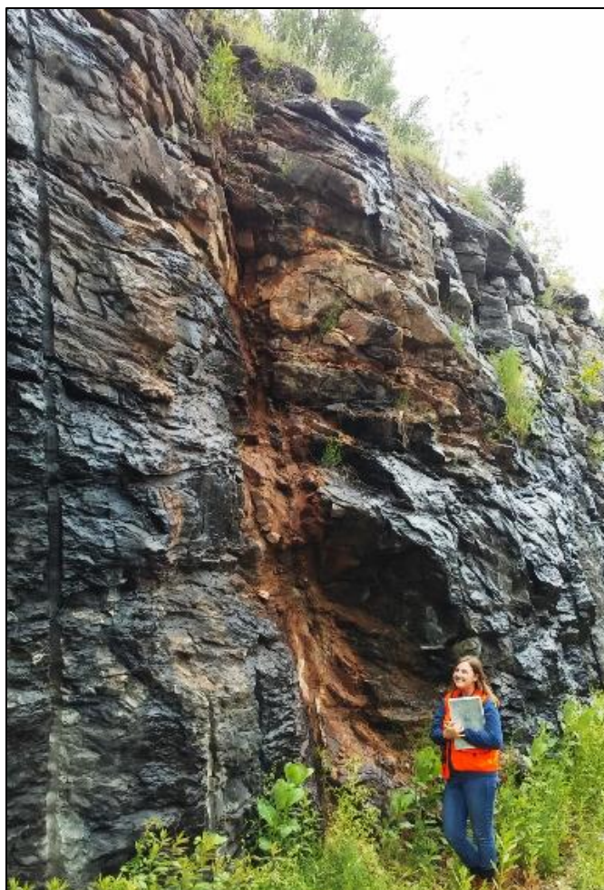
Madison in front of a rusty stained brittle normal fault zone that crosses Route 11 in Salem, CT
