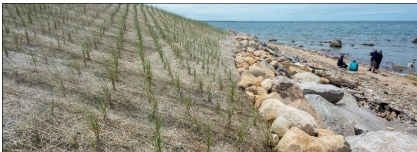
Figure 14. View facing the West Beach location after the revetment project in June of 2019. Boulders and native coastal grasses were strategically placed along the beach face to anchor sediment to prevent erosion. The RTK GPS and imaging setup is viewed on the right.
