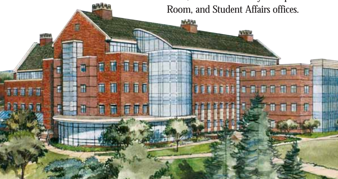
[top left] When completed in summer 2005, the Child and Family Development Resource Center will provide state-of-the-art early childhood instruction while supporting client families with comprehensive services; "The Great Room" will provide children with a multitude of learning activities.
