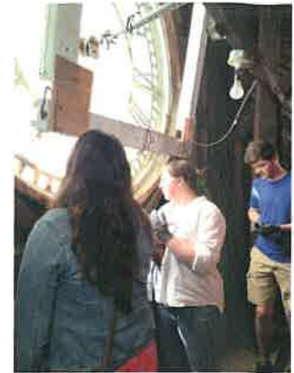
While also checking out the cool and creepy clock tower in the Town Hall!
