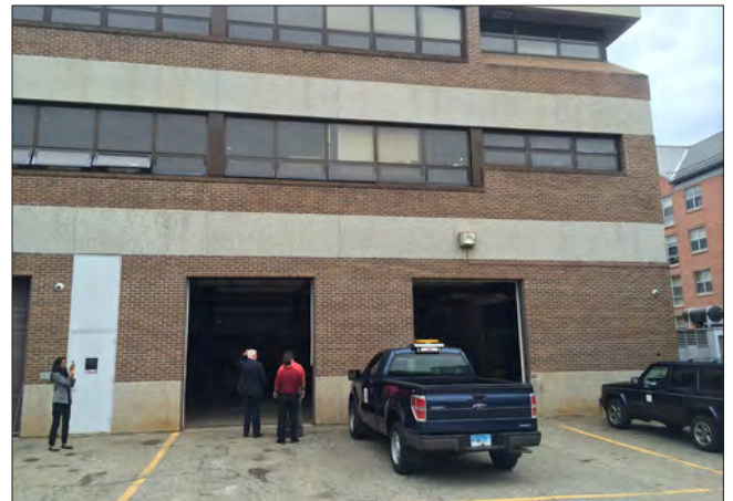
Facilities and Maintenance expansion site
