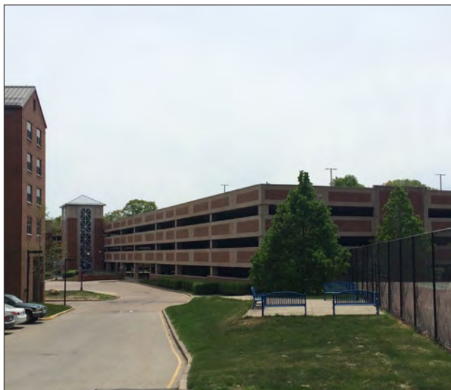
Cervantes Parking Garage
