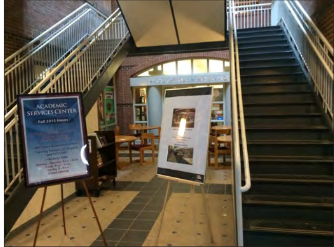
Ground level lobby with view to Library entry above blocked by stairs
